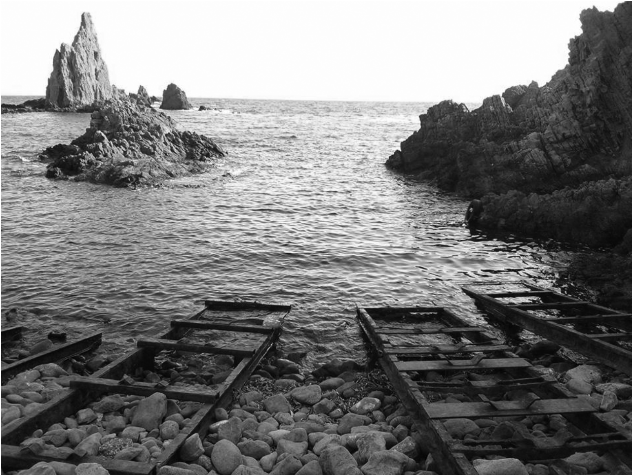
Figure 2.11. Traditional system for pulling in boats on stony ground. Arrecife de las Sirenas, Cabo de Gata. Almeria, Spain.
