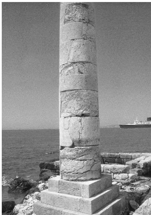
Figure 4.13. Column within the precinct of the so-called Tomb of Themistokles (Kantharos, n° 72). Reconstructed in 1952 from seven drums. Steinbauer 2000: 81.
