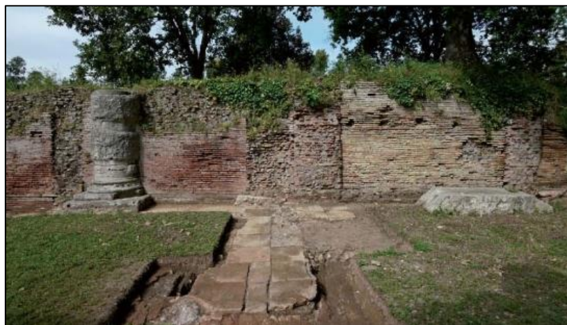
Figure 87: Warehouse facade wall (Bukowiecki et al. 2011, fig. 138)
