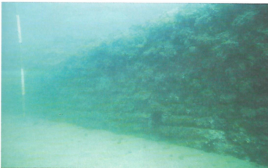
Figure 4. Antium harbour, Western dock, a brick-faced ruin on the seabed.
