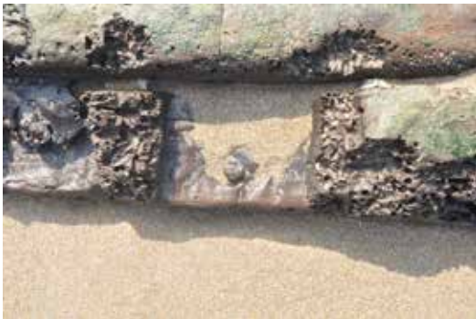
Figure 4.5 Mortise with a surviving portion of a peg in place
