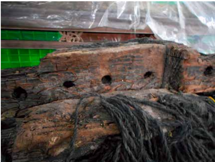
Figure 4.17 Holes of blind dowels at the longitudinal butt with hooked scarf joints
