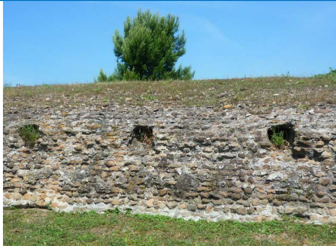
The emerging part of the North BW of Portus Claudius is made of concrete, which was probably cast in the way described by Bartoccini 13 .
