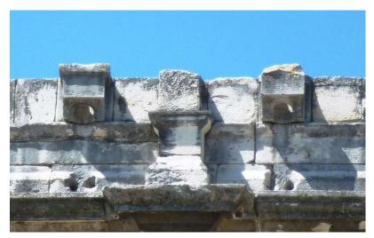
Feet of velum poles at Nimes. Note the mark of the poles on the wall and the clamp holes. (Photo A. de Graauw, 2011).
