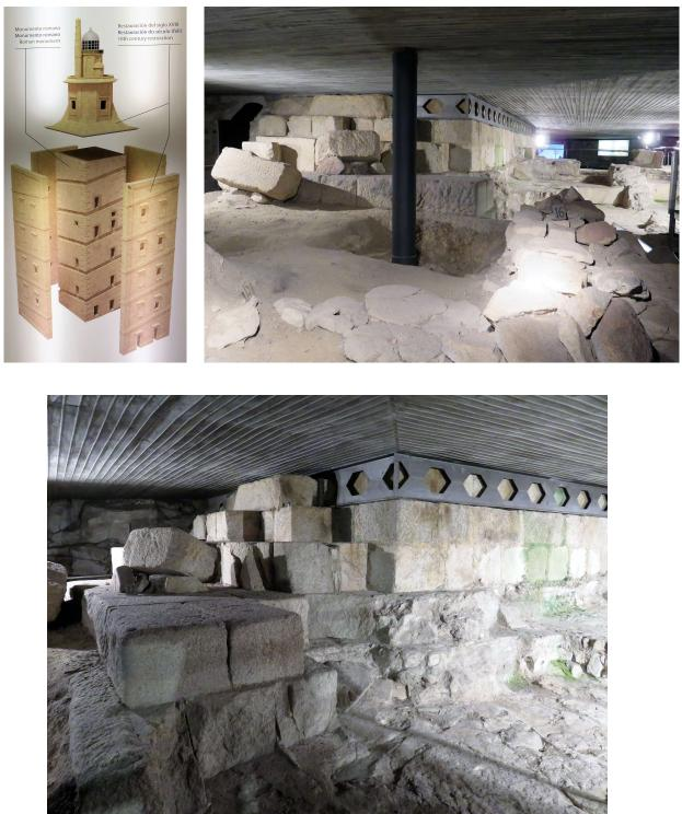
Tower of Hercules (A Coruna, Spain) showing reconstructed outer wall and ancient foundation level (A. de Graauw, 2017).
