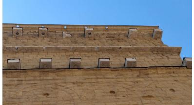
Feet of velum poles at Orange. Note the three superposed holes above the pedestal stone. (Photo A. de Graauw, 2020).
