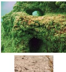
Belova's team in Alexandria<sup>139</sup>, reported a ca. 0.10 m hole near the edge of many large breakwater blocks ( $2 \times 2 \times 1 \text{ m}$ ). These holes have probably been used for ropes, either during construction of the structure, and/or for mooring ships later on.
