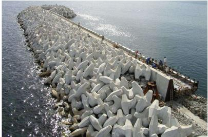
This picture (Fujairah) shows a modern BW under construction: large artificial blocks of concrete are used nowadays instead of rock, they are placed on top of, and as an armour layer of, a rubble mound made of quarry rock of several tons, which are themselves placed on a core made of quarry run. The crest structure (under construction) has a kind of "L" shape.
