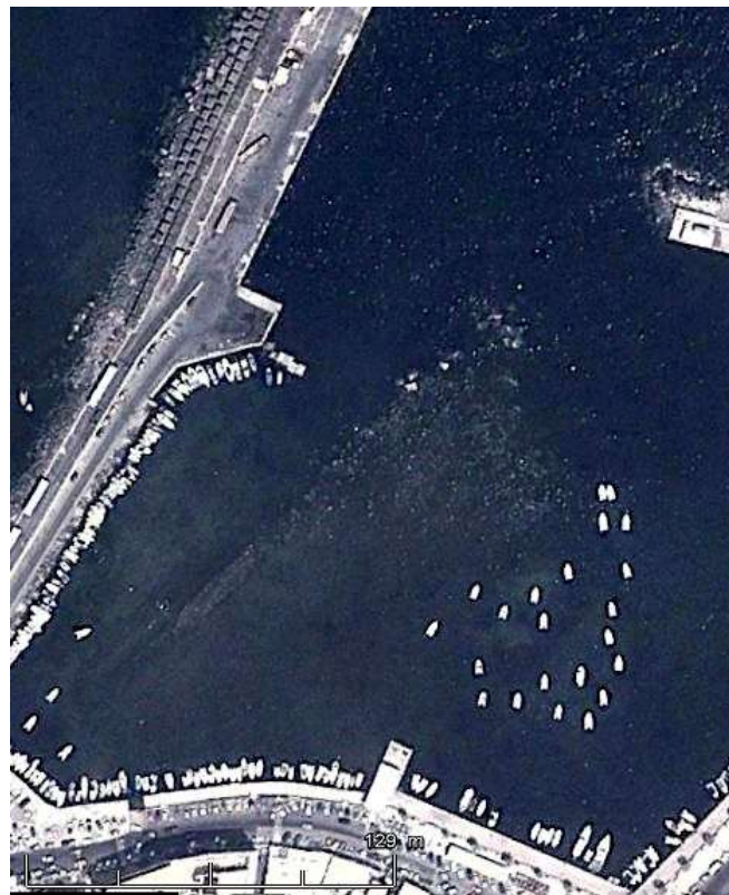
Kossura, GE 2012 (Pantelleria, Italy)
